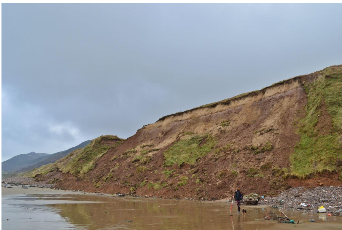
PI 13 Rossili Gower, cliff collapse adjacent to deserted medieval village
