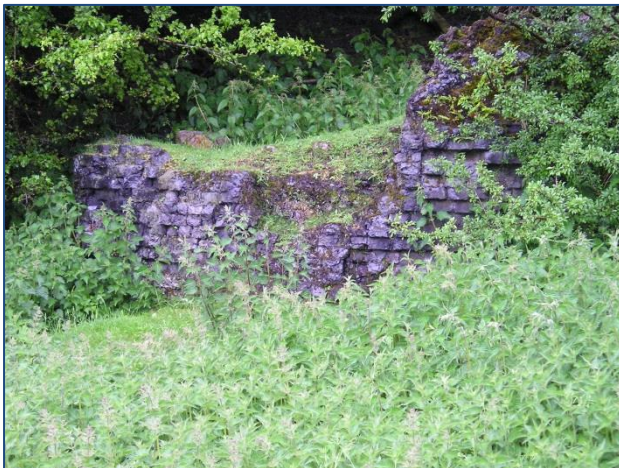
PI 1 Rhymney Union Ironworks upper furnace site
